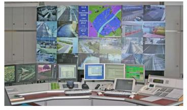
eyevis attached much importance on the possibility to use their cubes even in critical ambient light conditions or other challenging safety-related problems. The SXGA+ version uses a 1-chip-DLP<sup>®</sup> projector with a display resolution of **1400 x 1050 pixels**.
