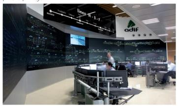
eyevis attached much importance on the possibility to use their cubes even in critical ambient light conditions or other challenging safety-related problems. The HD version uses a 1-chip-DLP® projector with a display resolution of 1920 x 1080 pixels.
