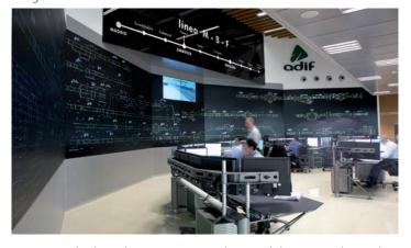
eyevis attached much importance on the possibility to use their cubes even in critical ambient light conditions or other challenging safety-related problems. The WXT version uses a 1-chip-DLP® projector with a display resolution of 1,920 x 1,200 pixels.
