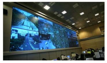
eyevis attached much importance on the possibility to use their cubes even in critical ambient light conditions or other challenging safety-related problems. The XGA version uses a 1-chip-DLP<sup>®</sup> projector with a display resolution of **1024 x 768 pixels**.
